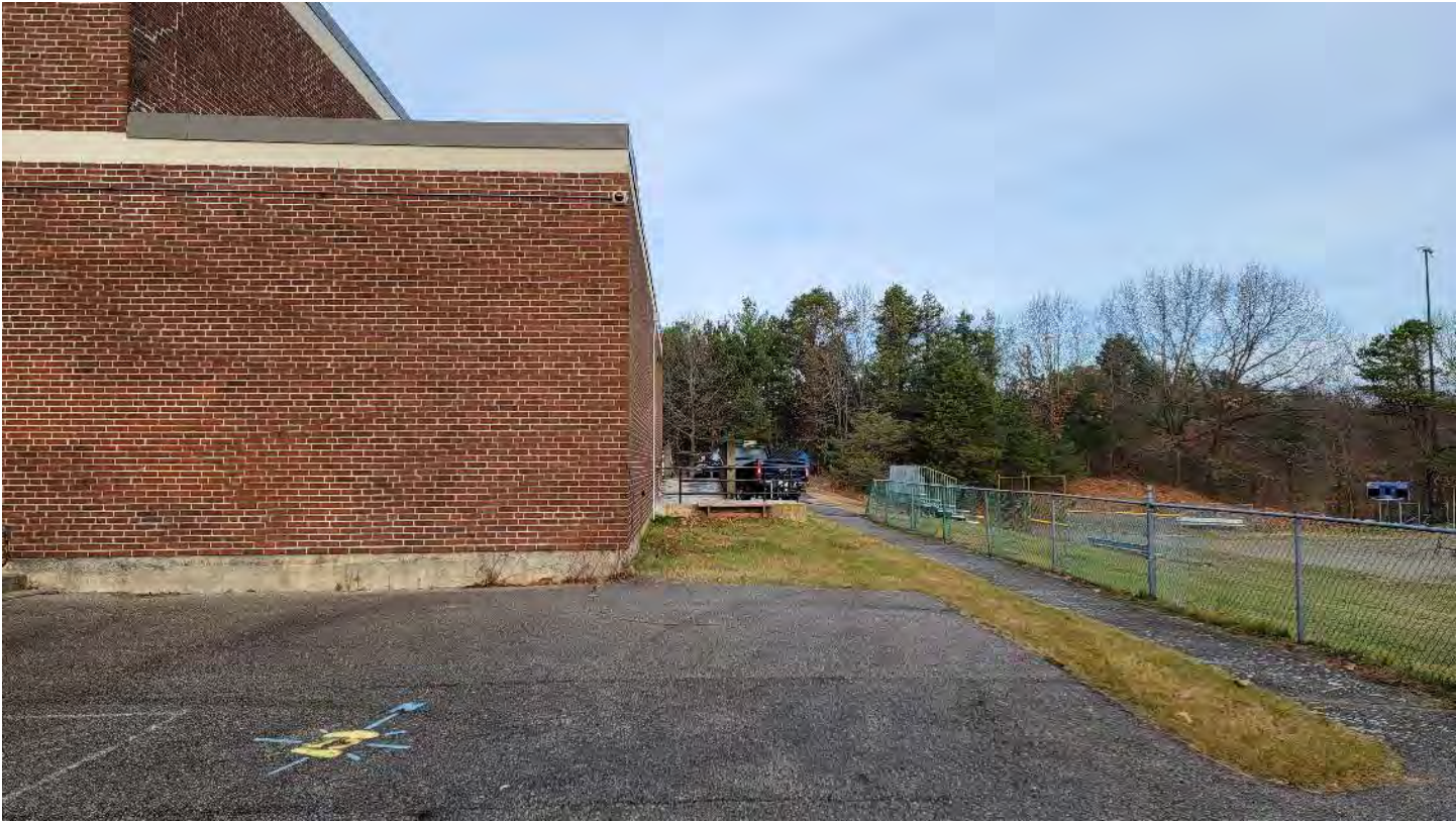
Rear of the subject building.
