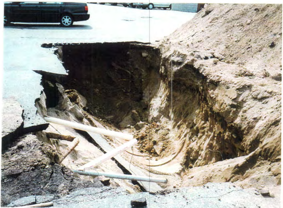
View of the excavation as seen looking southwest.
