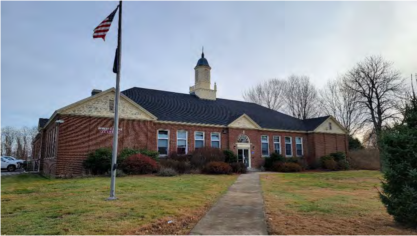
Front of the subject building.
