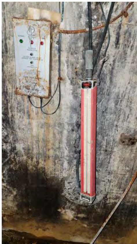
Tank guage to the former UST(s).
