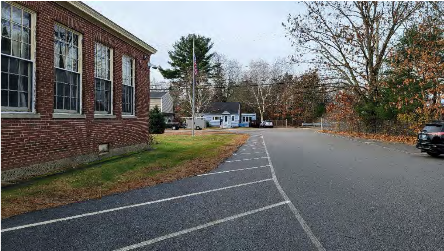
Northwestern side of the building.
