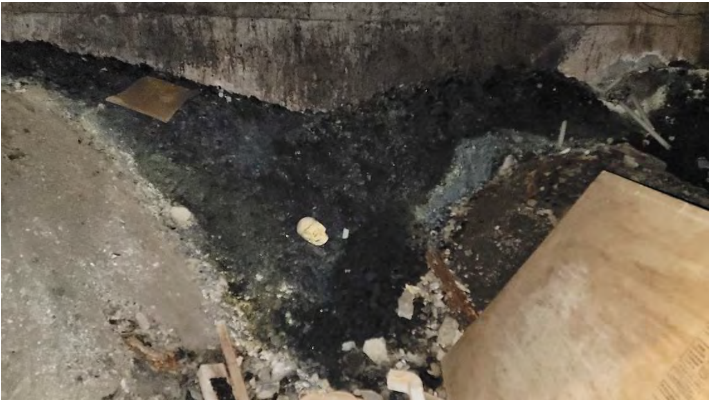
Remnants of historic coal storage.
