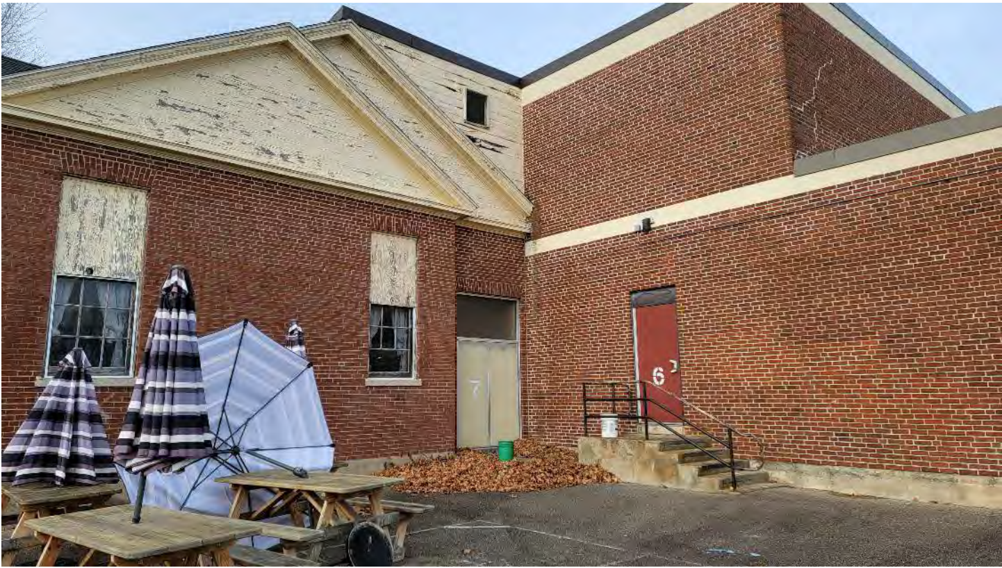
Rear of the subject building.
