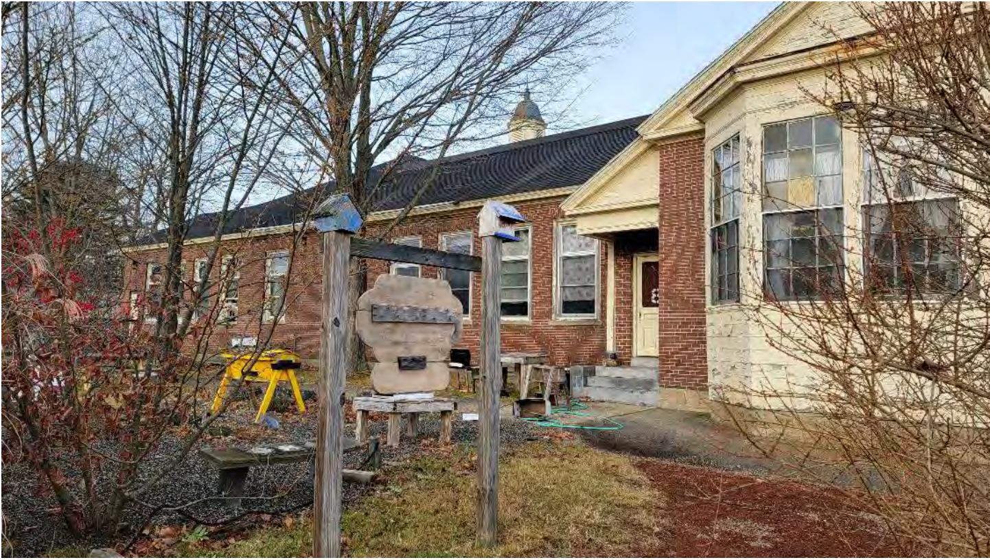
Southwestern side of the building.
