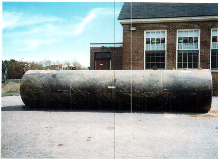
View of the UST after removal from the excavation.
