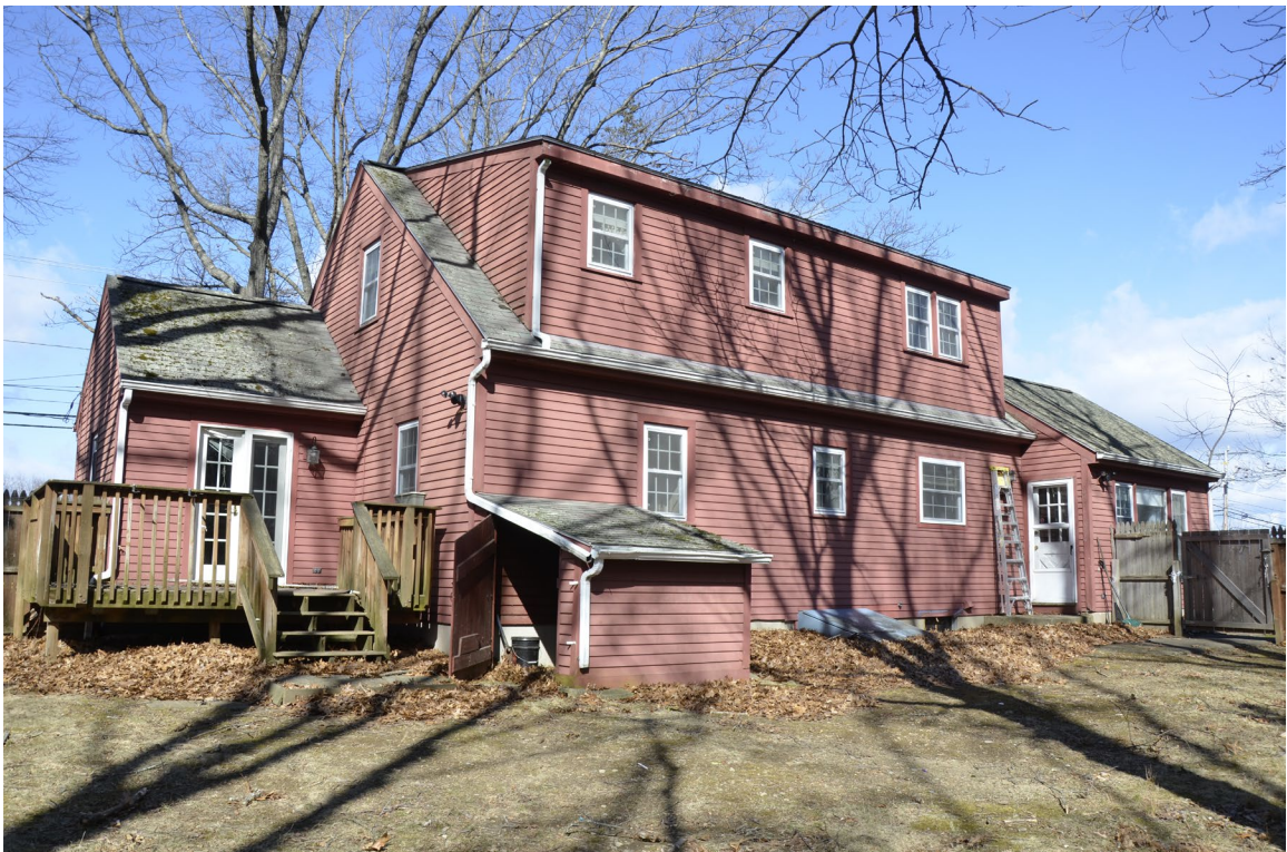
Photo 18) Rectory, rear elevation, facing northwest
