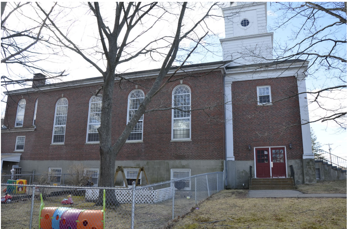
Photo 5) North elevation, facing south-southeast
