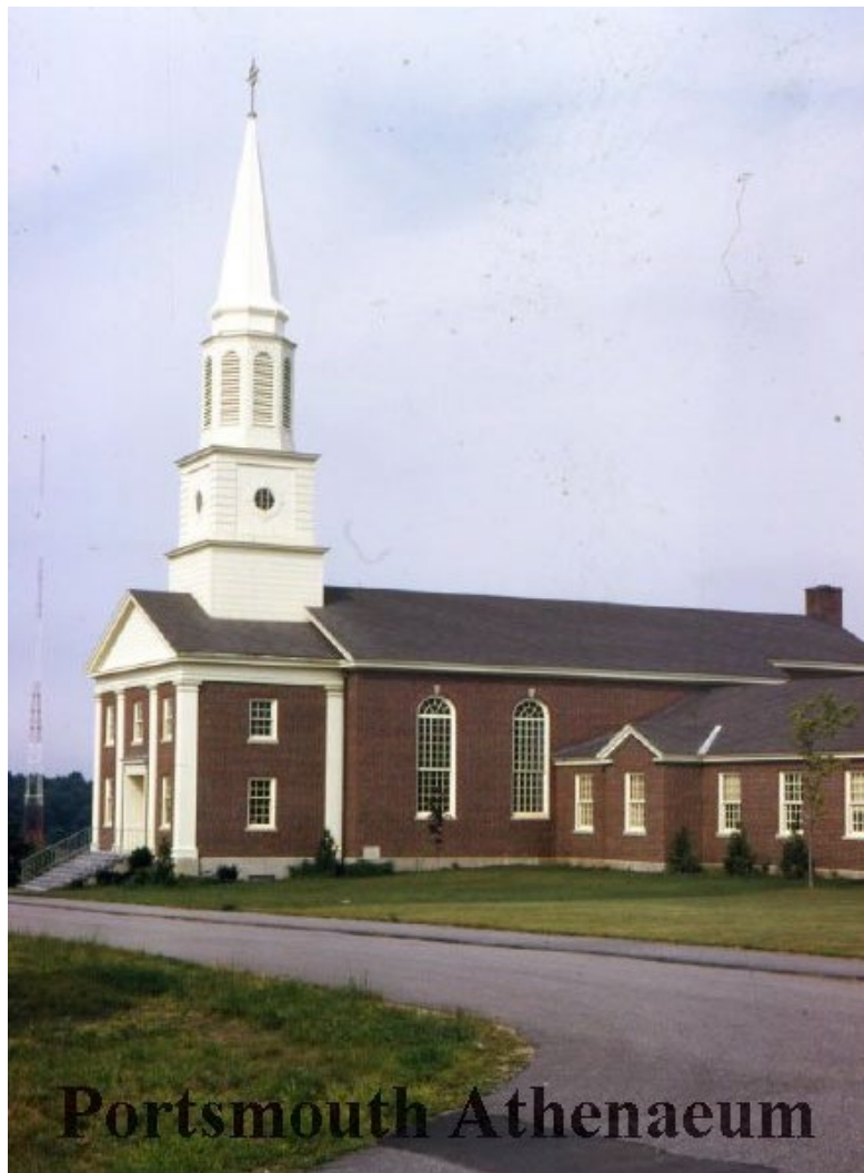
Figure 12: 1973 slide shows chapel before stained glass window installed (Portsmouth Athenaeum)
