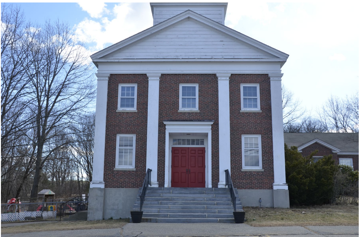
Photo 3) Façade detail, facing east-southeast
