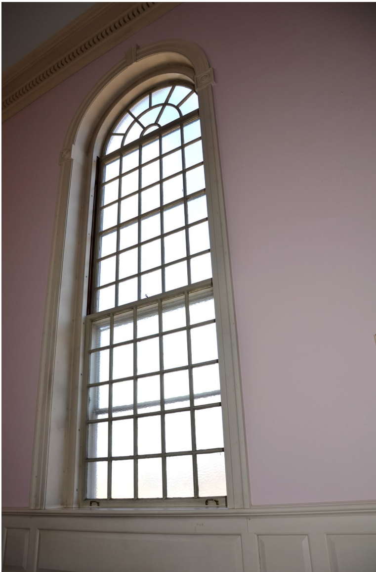
Photo 14) Interior window detail, facing northwest
