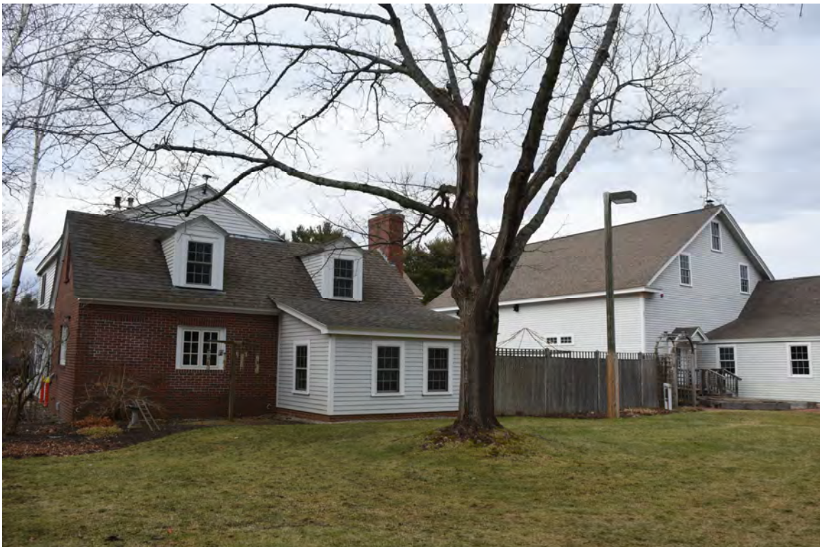
Photo 9) Caretaker's house and barn east elevations from front yard Reference (file name): PIC_9345
