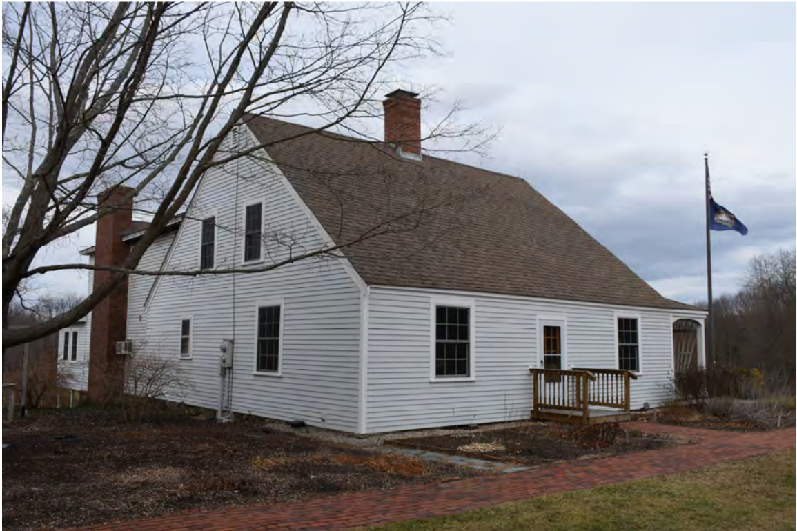
Photo 4) Cape west elevation and façade Reference (file name): PIC_9330
