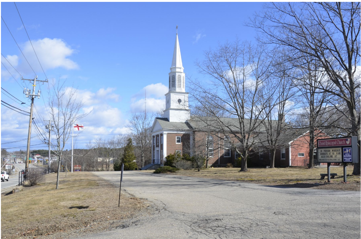
Photo 9) Southern entrance and driveway, sign, flagpole, facing northeast
