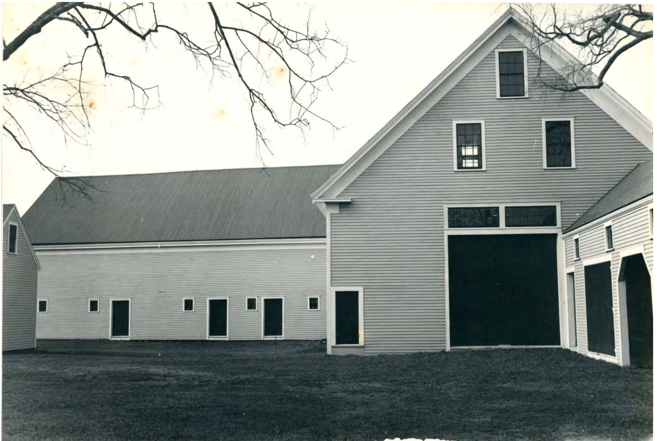
Figure 16. Outbuildings viewed from the back yard, facing west. Barn on site of John Elwyn Stone Forestry Learning Center at right, barn on site of maintenance barn at left (Courtesy of Alexander B. Warwick, Portsmouth Athenaeum)
