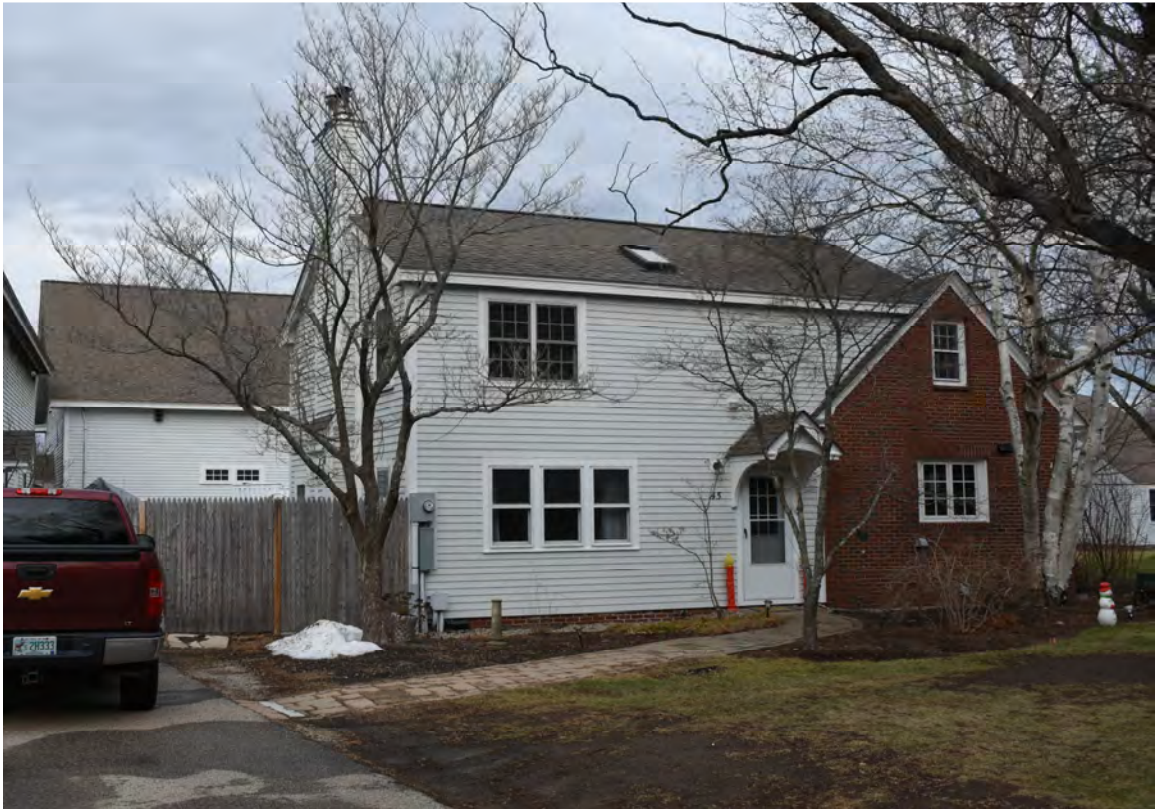
Photo 10) Caretaker's house south elevation from driveway Reference (file name): PIC_9348
