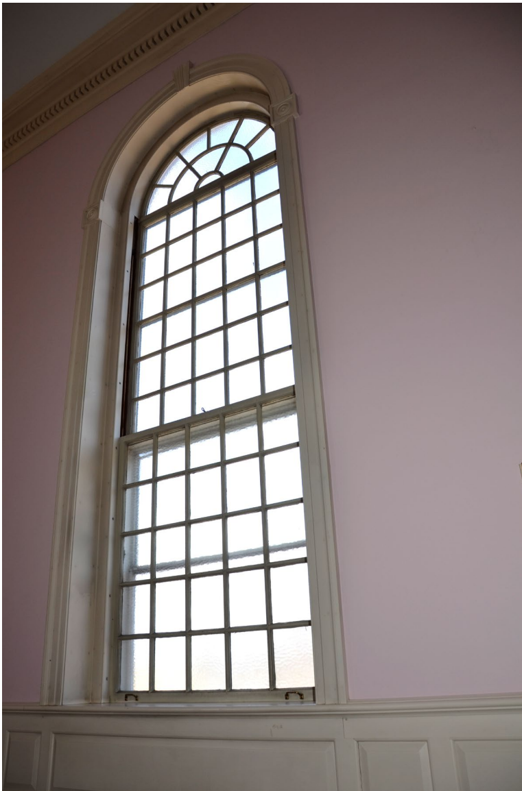
Photo 14) Interior window detail, facing northwest
