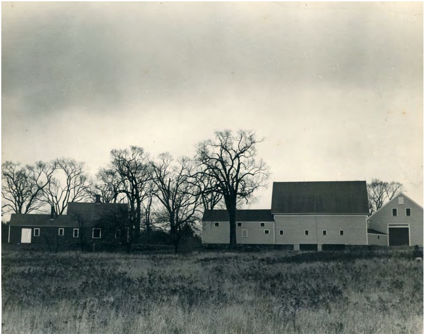
Figure 15. Rear (north) elevation of cape and barns, facing south from the field (Courtesy of Alexander B. Warwick, Portsmouth Athenaeum)
