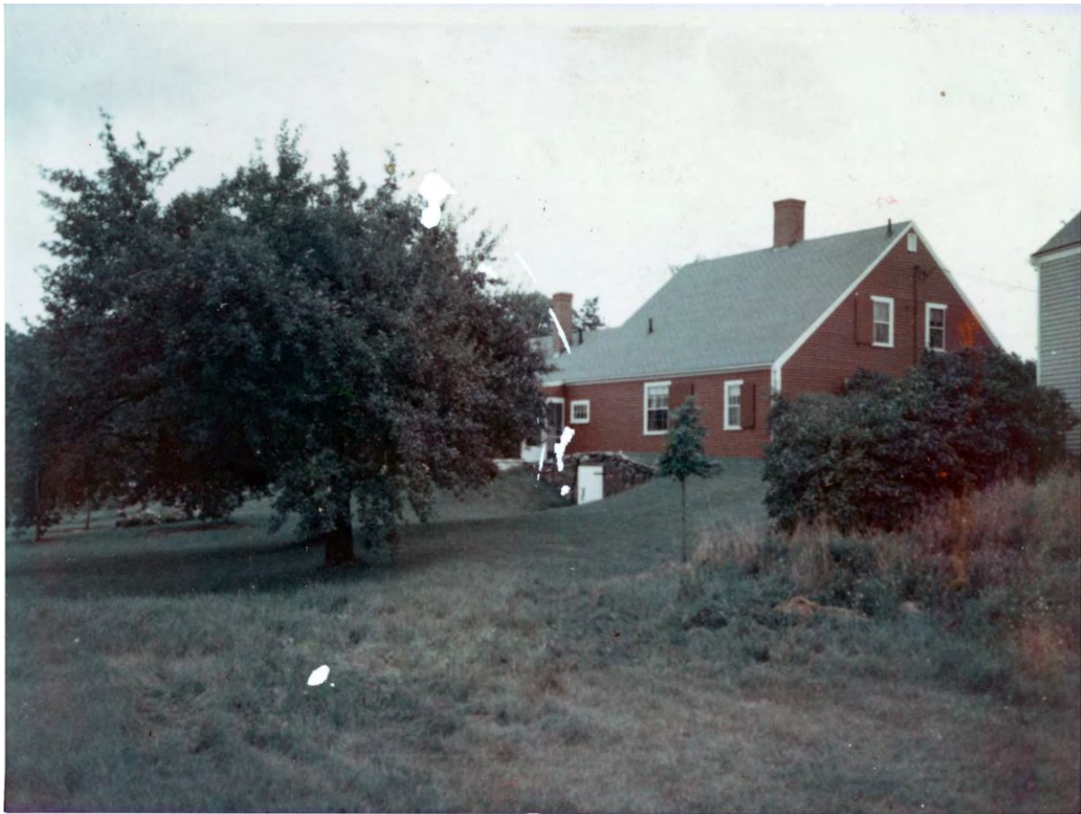
Figure 17. Rear of the cape, mid-twentieth century, facing southeast from the back yard (Courtesy of Alexander B. Warwick, Portsmouth Athenaeum)
