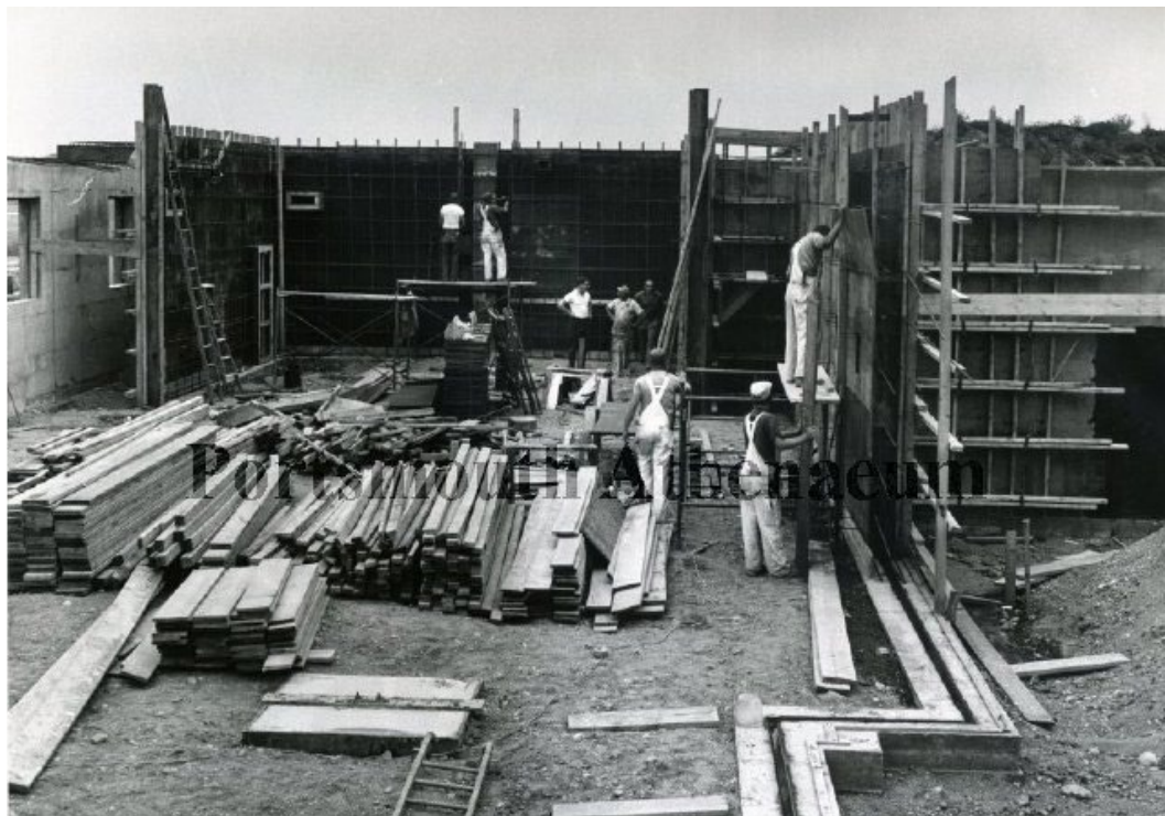
Figure 9: Foundation under construction 1965 (Portsmouth Athenaeum)
