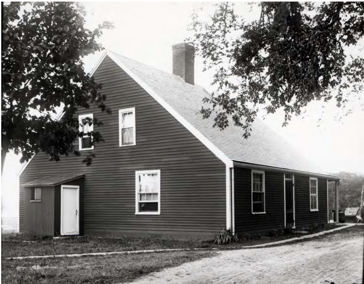
Figure 13. 1899 view of cape west elevation and facade, facing northeast (Courtesy of the Vincent D. Coyle Memorial Collection, Portsmouth Athenaeum)
