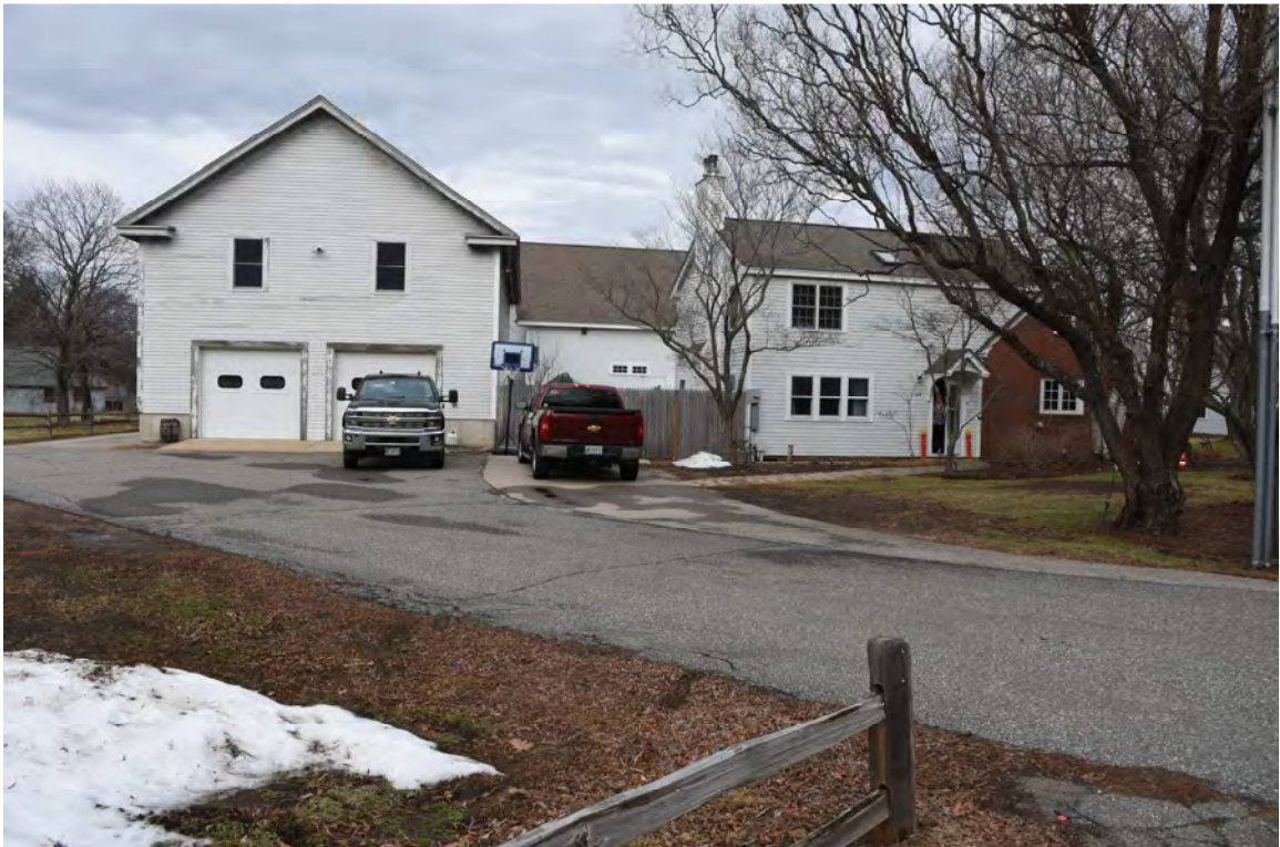
Photo 11) Maintenance barn and caretaker's house from driveway Reference (file name): PIC_9350
