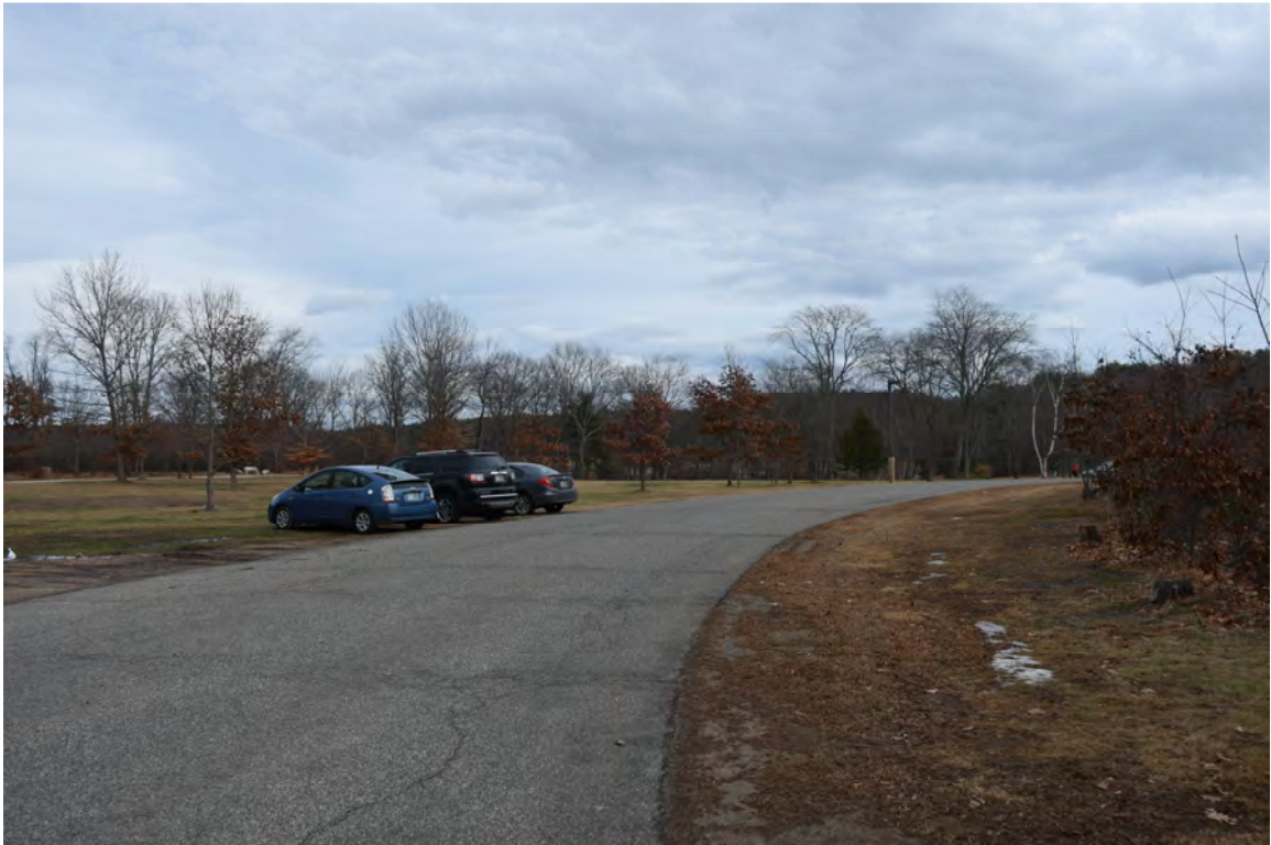
Photo 18) Driveway and parking lot Reference (file name): PIC_9370
