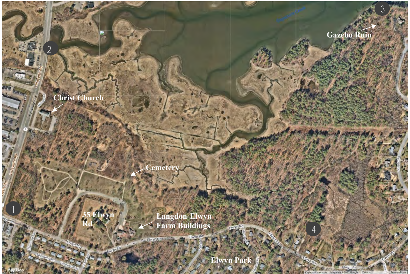
2021 Aerial photograph of the Urban Forestry Center via the City of Portsmouth's GIS mapping ( https://portsmouthnh.mapgeo.io/ )
