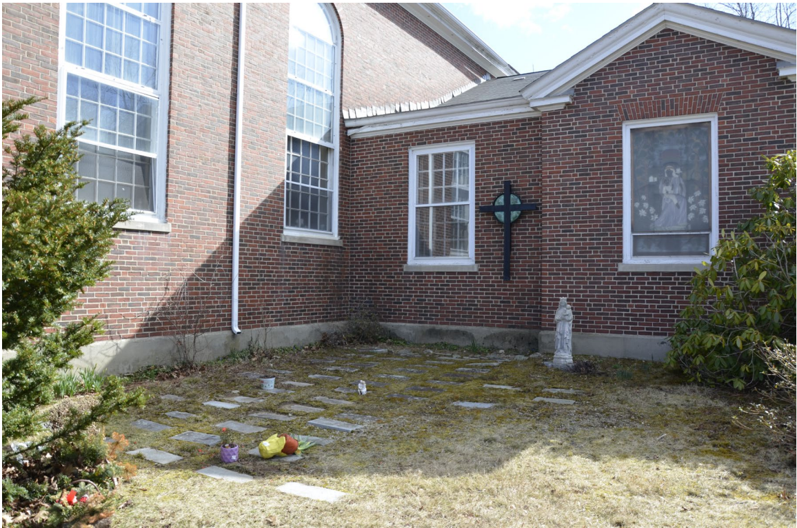
Photo 6) South elevation, chapel detail and memorial garden, facing east-northeast
